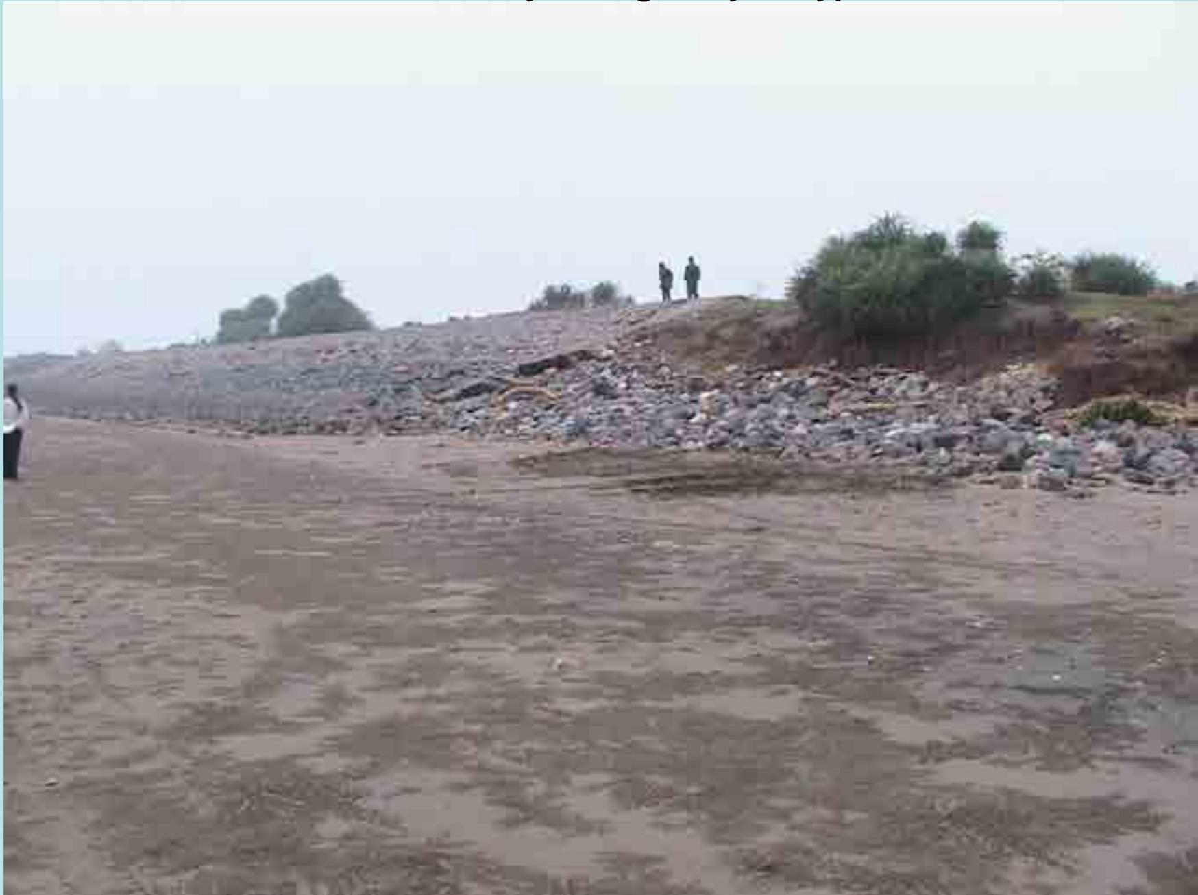
**On a badly eroded section of this dike, Vetiver provided some protection on the sea facing batter, but this was not enough to protect this dike during last year typhoon season, all washed away**
